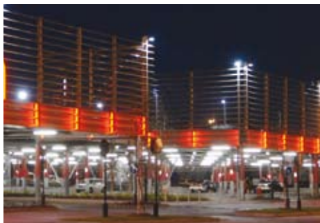
Parking Auchan Amiens (80) France Architecte: Richard Jacques Architecture Photo: ArcelorMittal - Claude Abron
