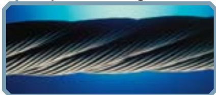
Suspension Bridge Cables
