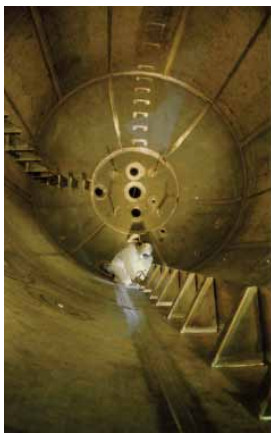
Welding solid alloy internals of a clad reactor.
