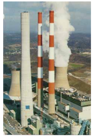
The new 1000-foot concrete chimney (left, foreground) at Allegheny Power System's Harrison Station, W. VA, contains three roll-bonded clad flues fabricated and erected by Graver Tank & Manufacturing of Houston, TX. This tower represents the largest application for roll bonded clad in the power generation market at the time.
