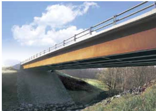
Steel bridges in the U.S.A. are increasingly using new high performance steels (HPS 50W, HPS 70W, HPS 100W) produced by Arcelor-Mittal USA with Finline practices for improved toughness.
