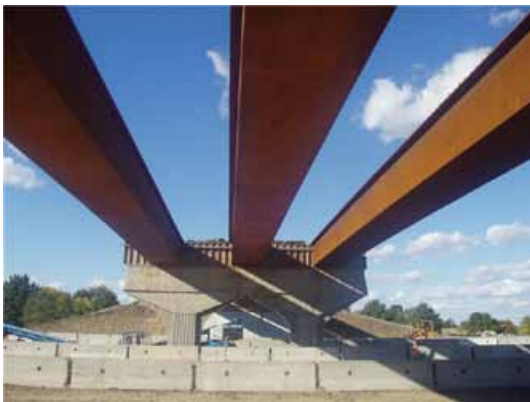
HPS 100W bridge in Nebraska. Photo: Professor Atorod Azizinamini
