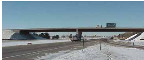
HPS 100W bridge in Nebraska Photo: Professor Atorod Azizinamini
