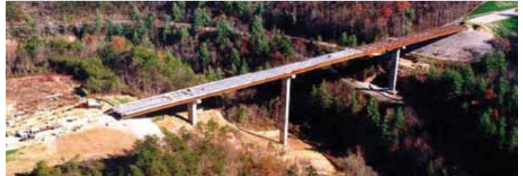
Clear Fork Creek Bridge in Tennessee
