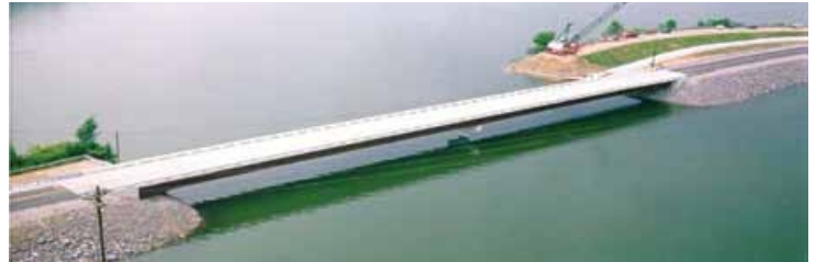
Martin's Creek Bridge in Tennessee
