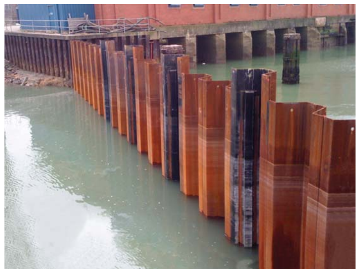
Fig. 13 Port of Shoreham. AMLoCor steel sheet pile wall
