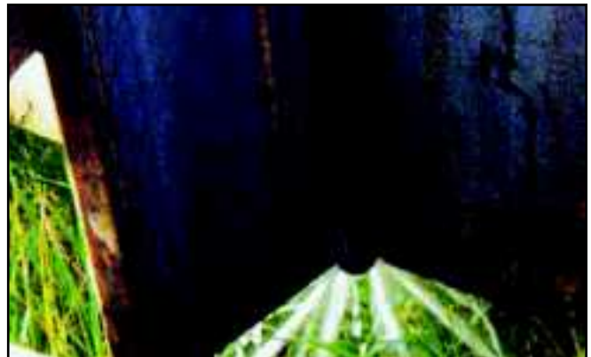
Photo 1: Toe of U sheet pile with two jets in action
