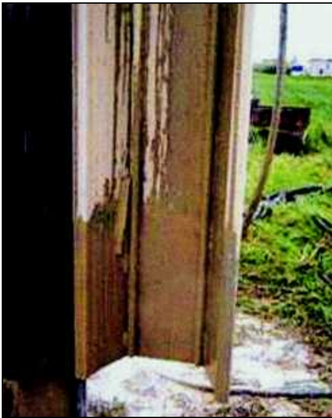
Photo 2: Extracting jetted U pile
