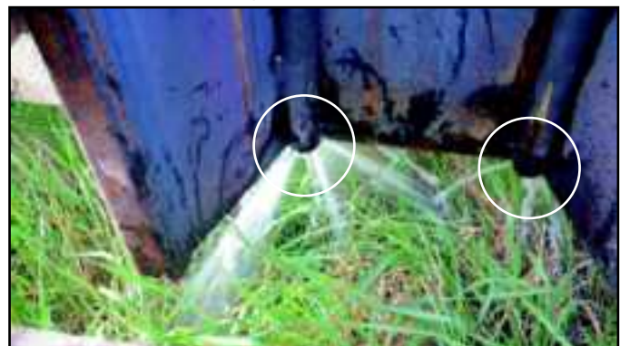
The jetting pipe ends flush with the toe of the sheet pile.
