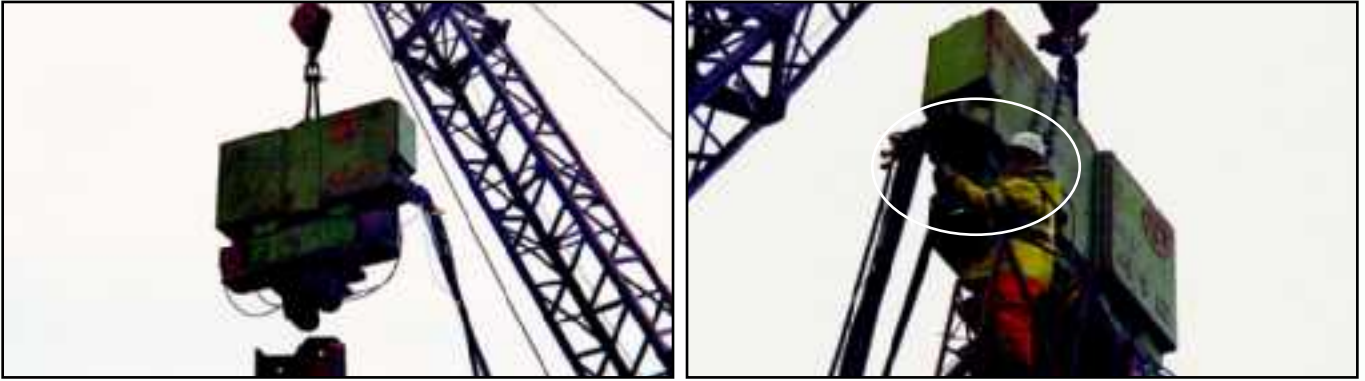
Hoses and jetting pipes being connected.
