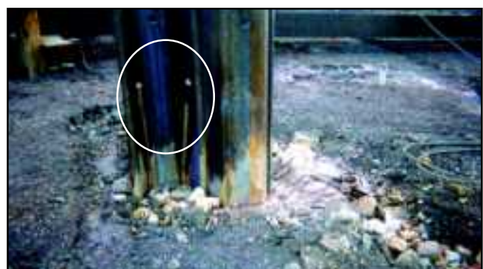
The top of the jetting pipe may be bent to facilitate connection of the supply hose.
