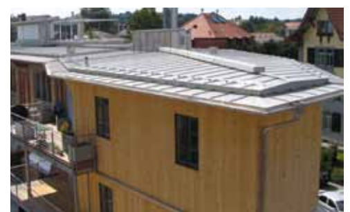
Alte Kohlenhandlung, Langenthal – Switzerland. Architects: Blum & Rossenbacher Executed using grade UGINOX FTE
