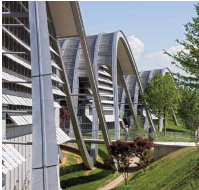
entrum Paul Klee, Suisse Renzo Piano Building workshop In collaboration with ARB (Bern) © RPBW – Michel Denancé Achieved with grades 304, 316L UGITOP finish
